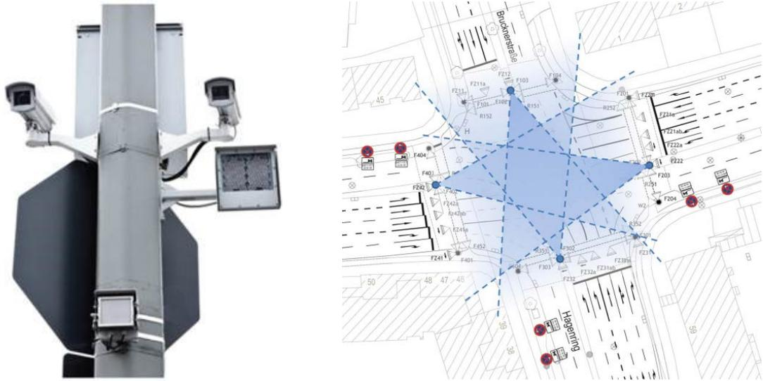
Figure 2: Single pole installation of MSS (left) and bird's eye view of all sensor locations (right) In addition, SENV is installed on the Western and Southern pedestrian crossing. There are four installations which are respectively attached on the opposite sides of the crossings. Each of these installations consists of a stereo camera system and an infrared lighting unit.
