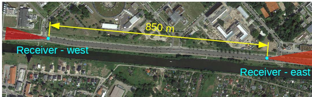
Figure 1: UTRaLab and its two gantries.
