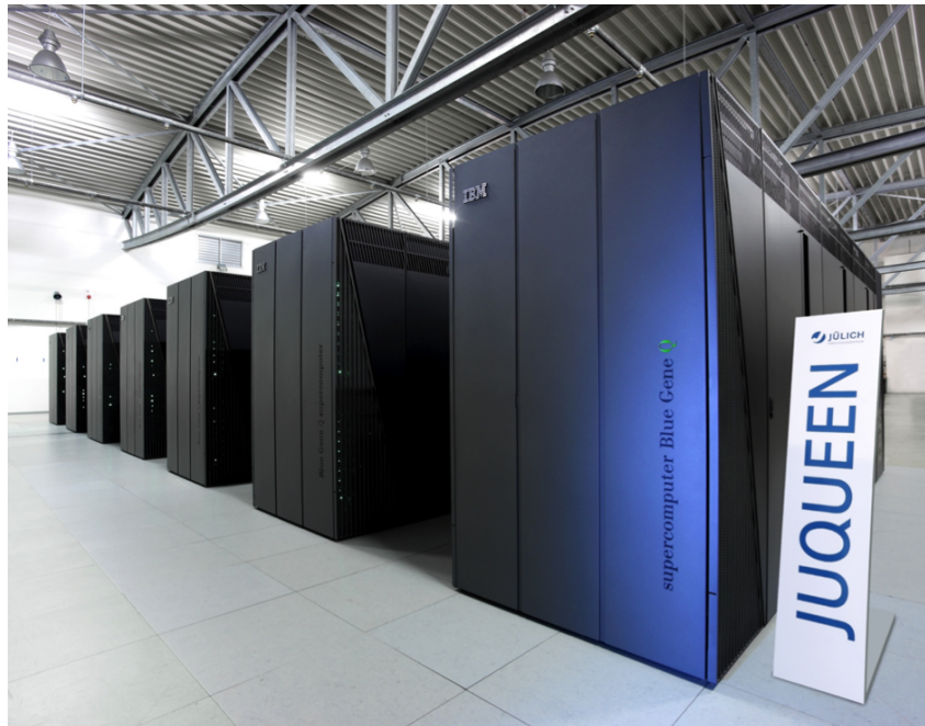
Figure 1: JUQUEEN at the Jülich Supercomputing Center.
